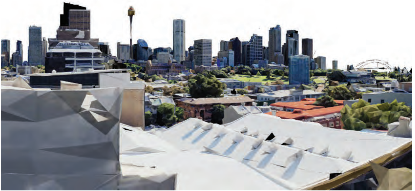
Viewpoint 45: Original Site Photo - including Metromap 3D LIDAR survey overlay.
